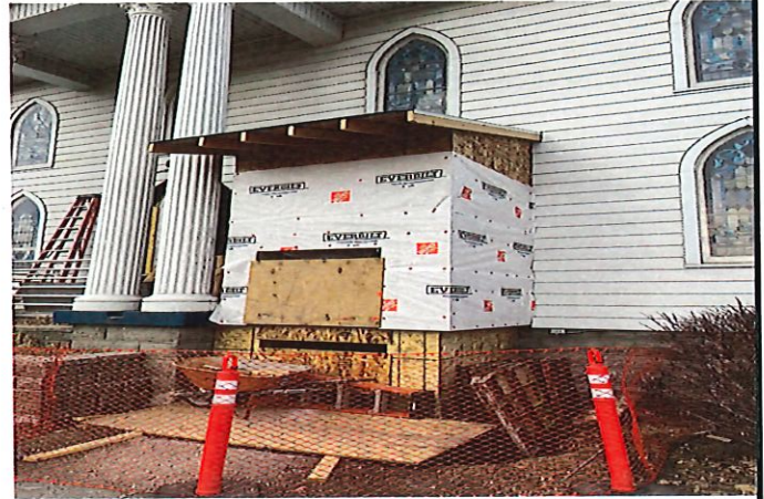
Close up view of the continued lift construction
