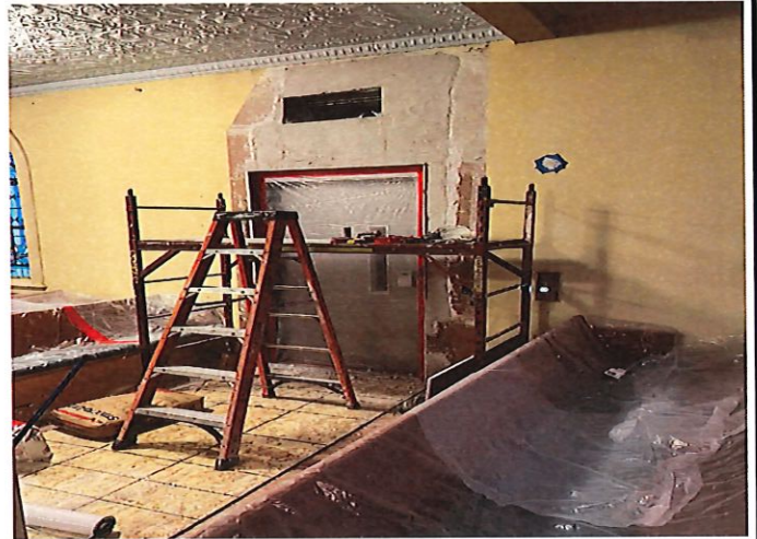
Inside view of the lift installation and finishing work to be completed
